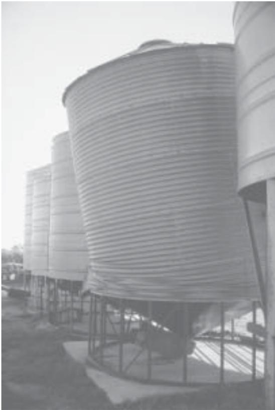
*Figure 2. Silo distorted when outloading lupins.*
