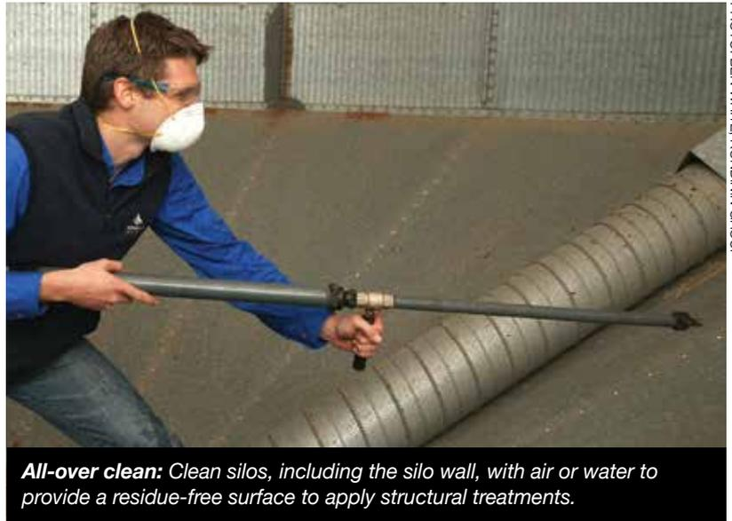
**All-over clean:** Clean silos, including the silo wall, with air or water to provide a residue-free surface to apply structural treatments.
