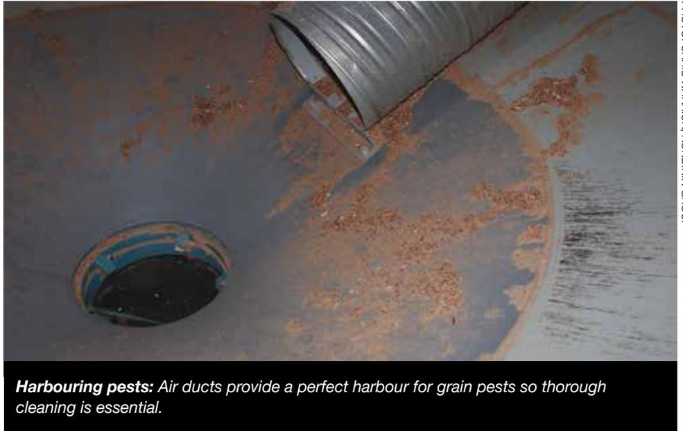
**Harbouring pests:** Air ducts provide a perfect harbour for grain pests so thorough cleaning is essential.
