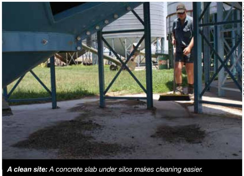
**A clean site:** A concrete slab under silos makes cleaning easier.
