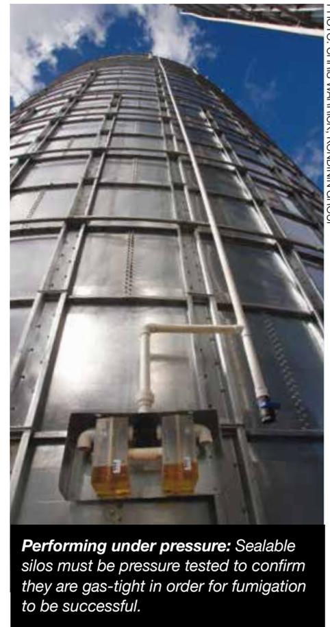
**Performing under pressure:** Sealable silos must be pressure tested to confirm they are gas-tight in order for fumigation to be successful.
